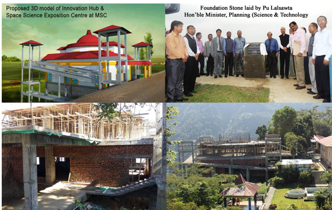
Construction of Innovation Hub and 8.0M Diameter Dome Planetarium
